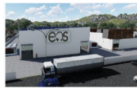
PowerHouse (10MW = .15 acres) (1)
