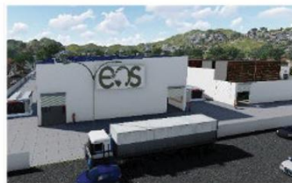
PowerHouse (10MW = .15 acres) (1)
