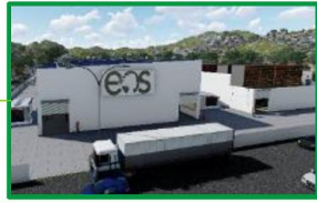
Containerized Power House
