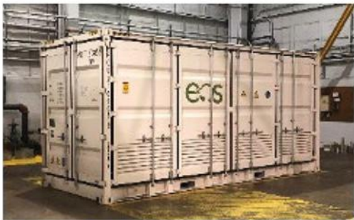
Containerized (10MW = 0.5 acres)
