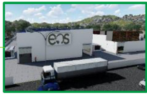
Containerized Power House
