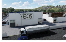
PowerHouse (10MW = .15 acres) (1)
